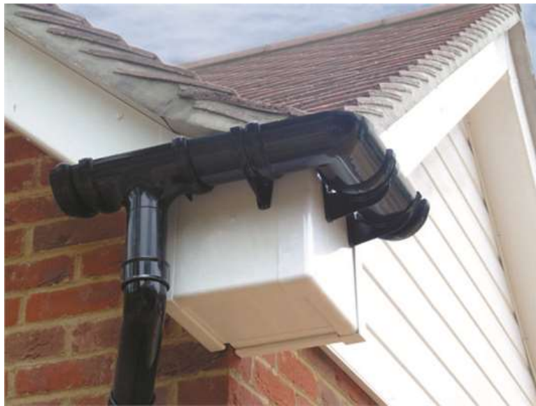
Figure 4 – gutters and downpipes
